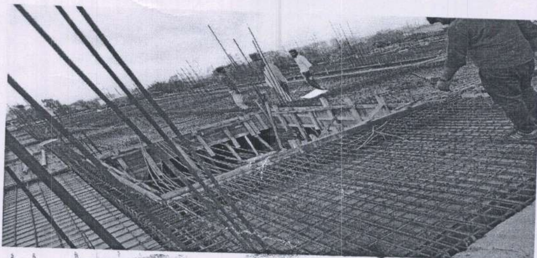
Fig 4: Footing reinforcement
