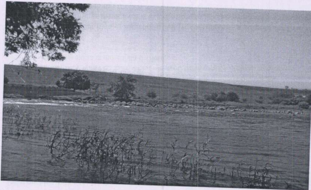
Fig. (c) Chandoli Dam Upstream side
