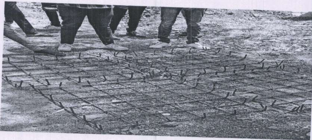
Fig 4: Footing reinforcement
